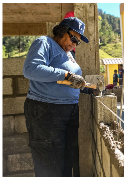
LeSesne installs bricks for the new addition
